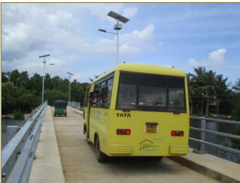
Eliya Tuck-Tuck and Eliya School bus at the new bridge
